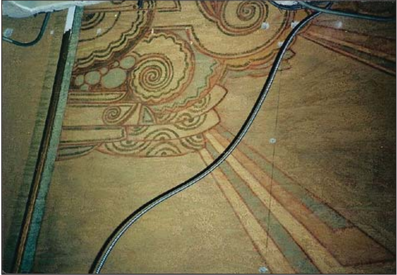
Detail view of finishes at ceiling of lobby prior to 1998 renovation. (Source: Gary Parks, 1998, http://www.flickr.com/photos/howardbhaas/285871917/ ).
