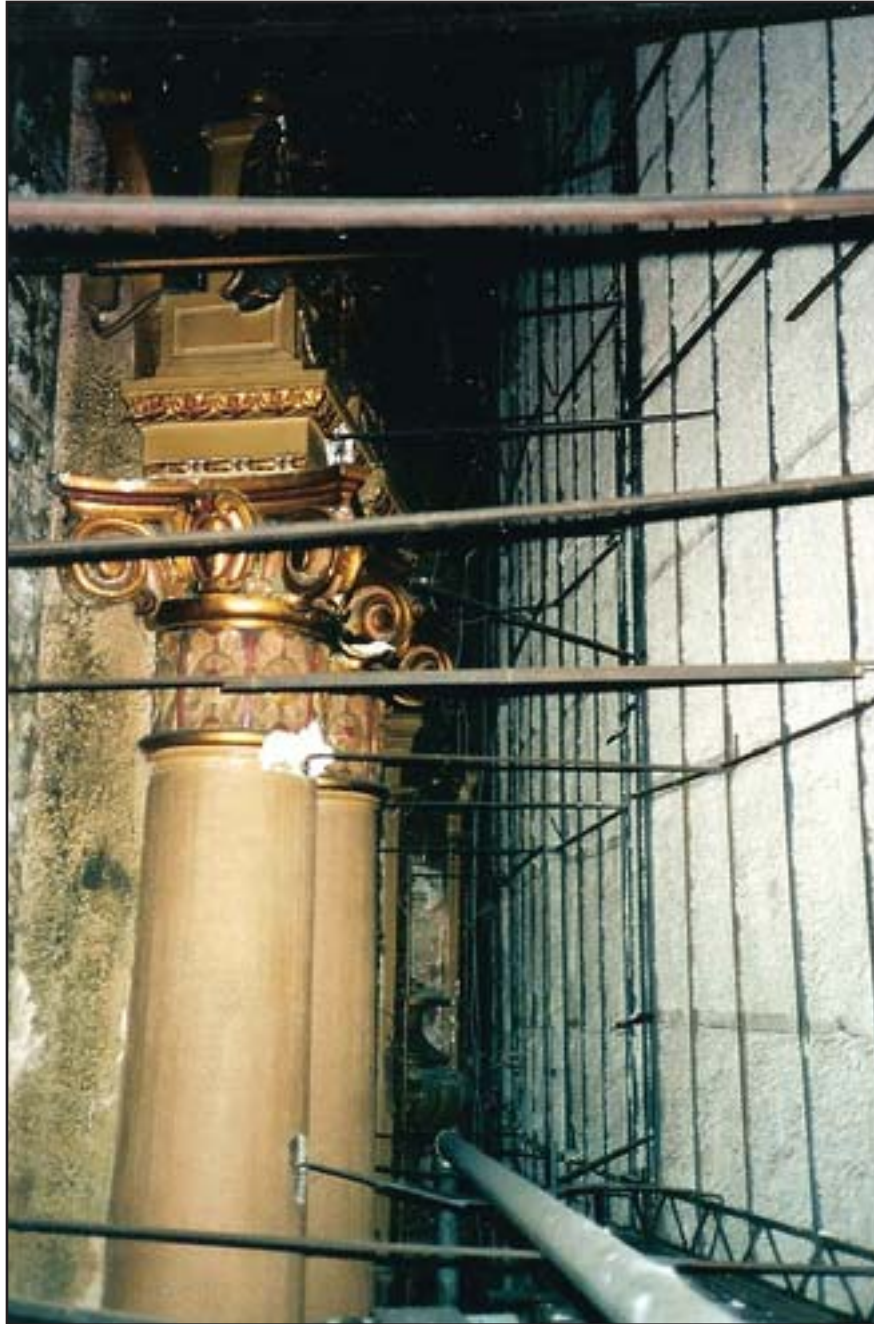
View of original 1924 Ionic columns in auditorium behind 1941 renovations prior to 1998 renovation. (Source: Gary Park, 1998, http://www.flickr.com/photos/howardbhaas/285871917/ ).
