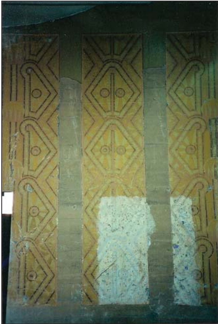
Detail view of finishes at lobby wall prior to 1998 renovation. (Source: Gary Parks, 1998, http://www.flickr.com/photos/howardbhaas/285871917/ ).
